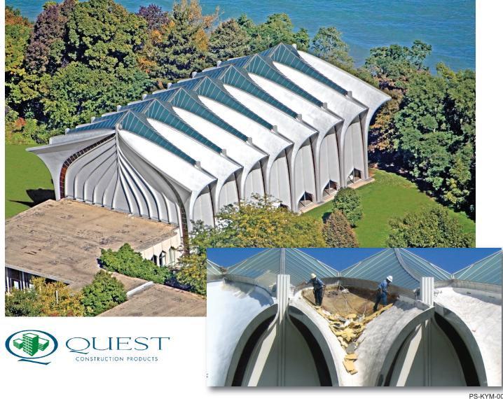
Before IRC could apply any new materials they had to remove the old roofing system. After the old materials were removed and the building's concrete roof deck was exposed and cleaned, they began applying the new BASF foam system.
